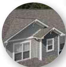
Roofing and Ventilation
